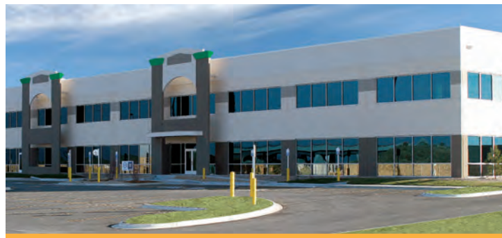
General Motor's Service Parts Distribution Center located in ProLogis Park 70, Completed November 2003
